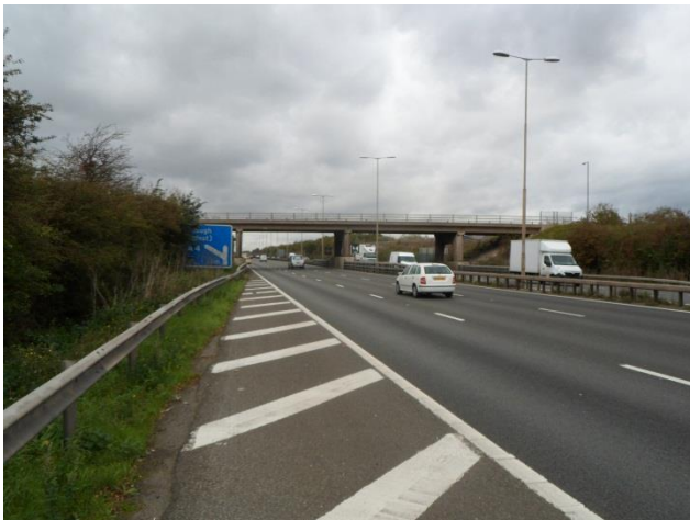
Figure 3 Typical existing overbridge with discontinuous hard-shoulder
