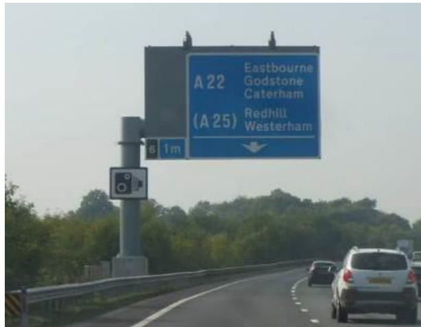
Figure 8 Typical sign-only cantilever gantry (one leg)
