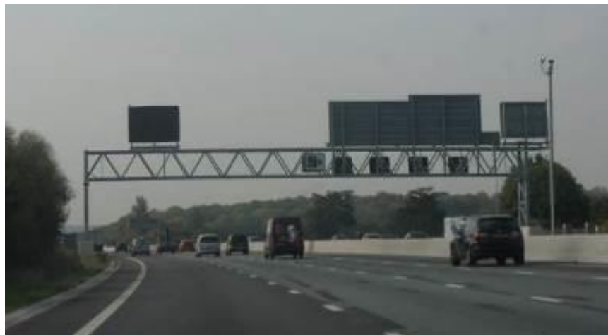
Figure 11 Typical super-span portal gantry
