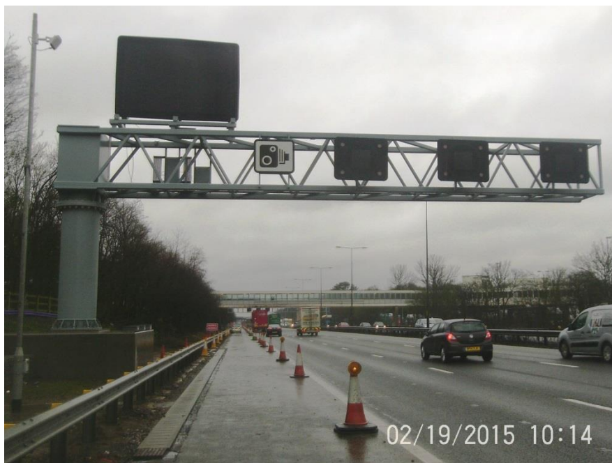
Figure 9 Typical super cantilever gantry
