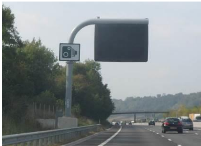
Figure 4 A cantilever gantry solely supporting an MS4 over lane 1
